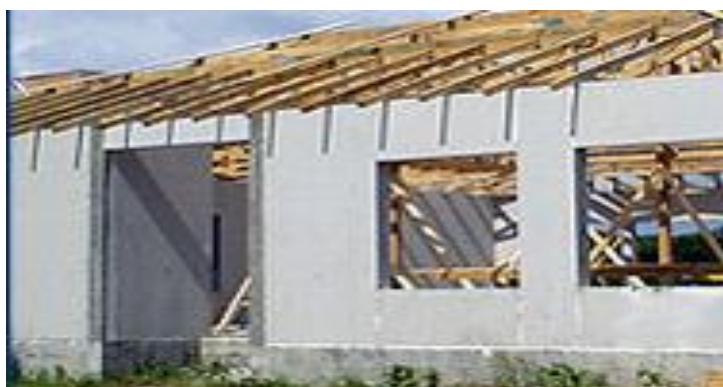
Figure 17. A residential home with concrete walls.
