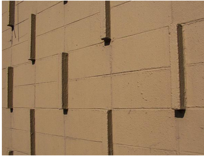
Figure 19. Close-up of Rodeway Inn cinder block external wall.
