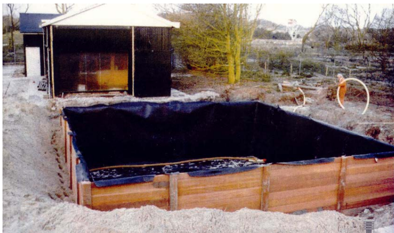
Figure 4. Sand box under construction
