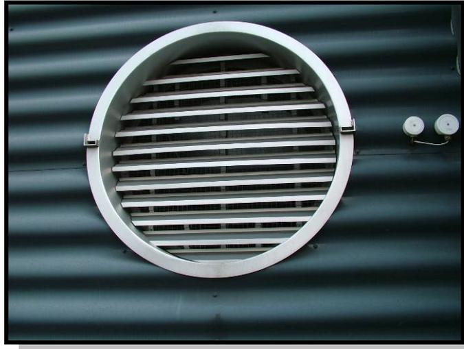
**Figure 6. Close-up of air vent on tower, which could be a point of entry in the GHz frequency regime.**
